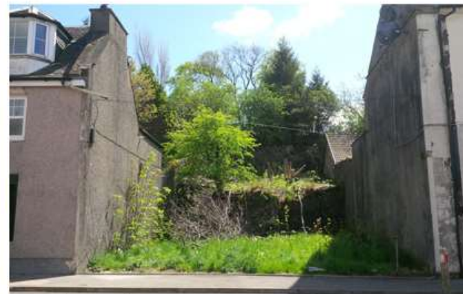
vacant gap site
