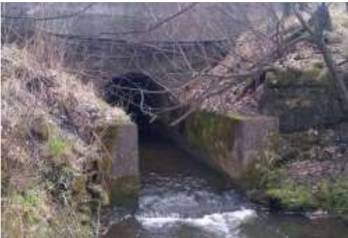
culvert to stinky point
